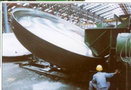
Design, Fabrication & Installation for the whole equipment 整套設備之材料, 製造, 安裝
