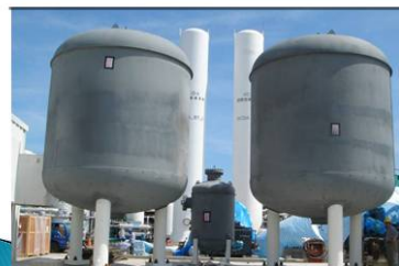
Molecular Sieve Adsorber
