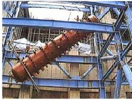
Steam drum installation 汽鼓安裝
